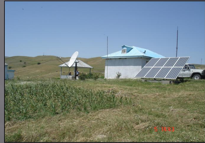
Telemetric seismic stations
