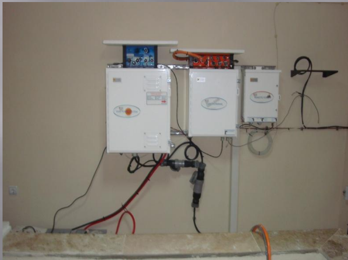
Inside view of seismic station
