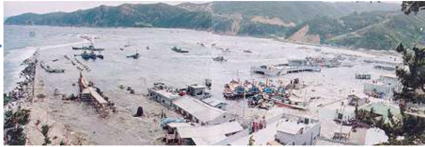
Damage of Tsunami(Imwon port)
